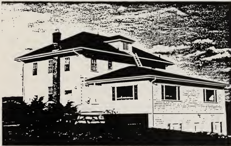
NEED Collaborative - Tract #17-2710 Bldg #T-116
